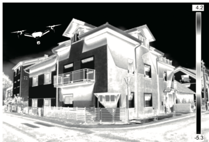
Figure 14 Thermal Imaging using a Drone
