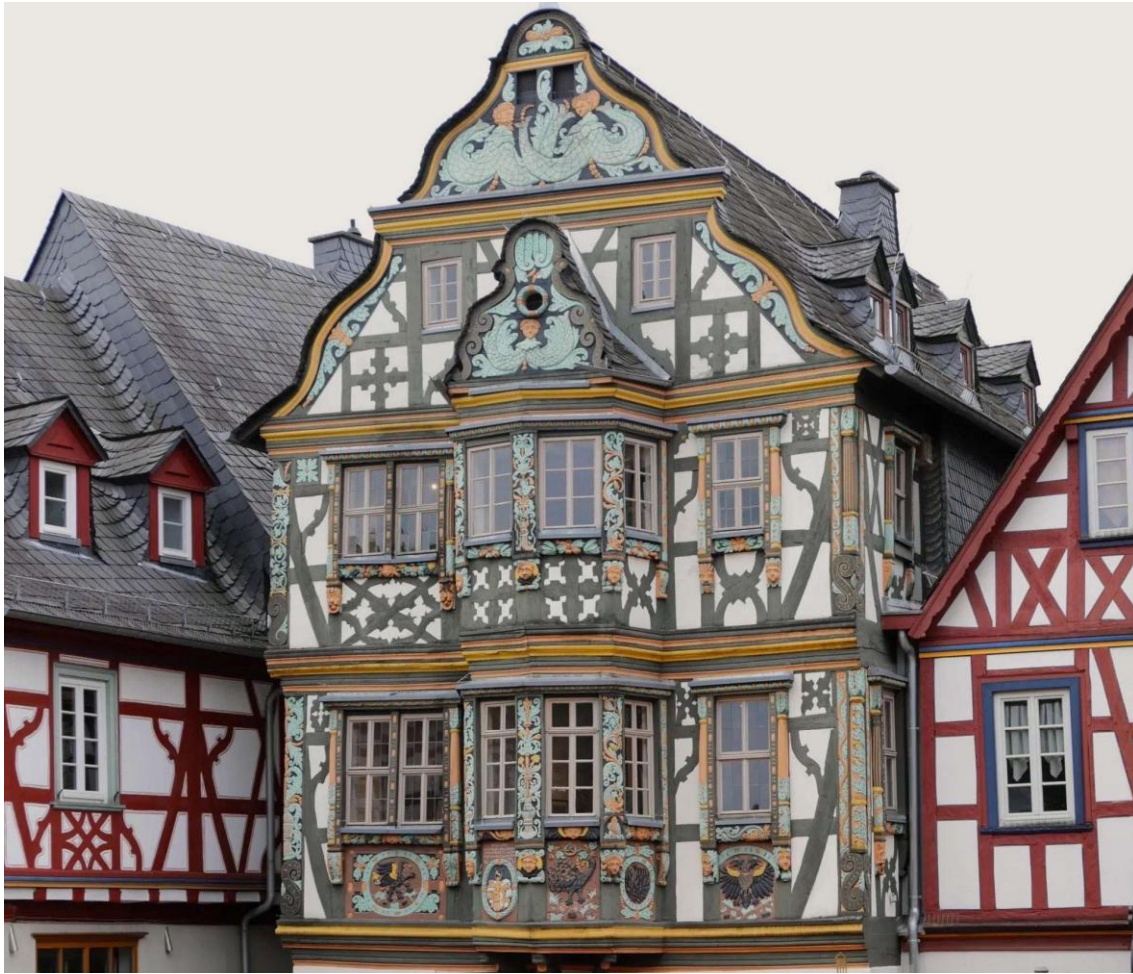
Figure 3.2 – Evolution of timber structural systems: Half-timbered construction (Fachwerk) as developed in Central Europe, illustrating the structural role of the timber skeleton and its long-term durability.
