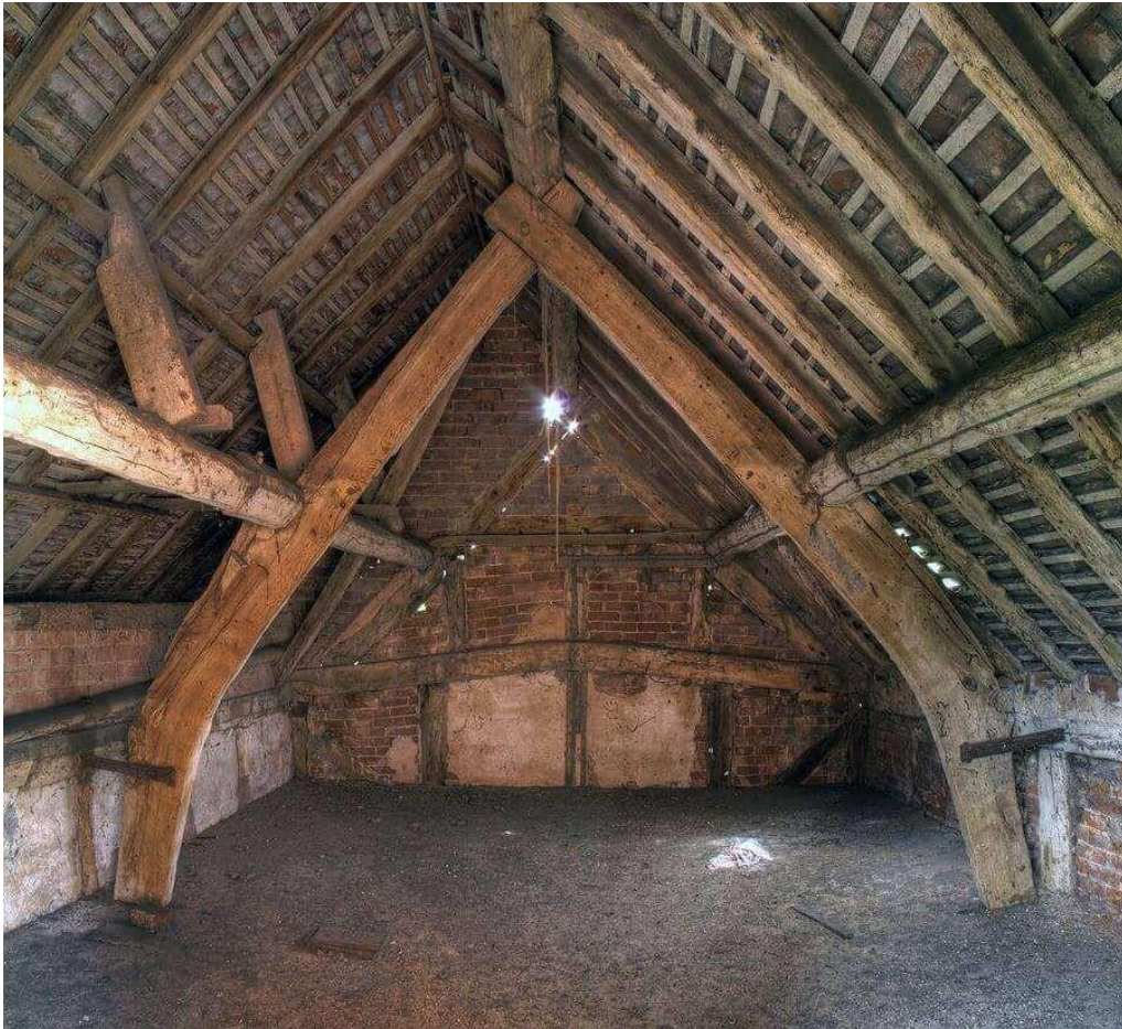
Figure 3.1— Evolution of timber structural systems: Traditional timber framing systems in medieval Europe, characterised by load-bearing wooden frames combined with infill materials such as masonry or adobe.
