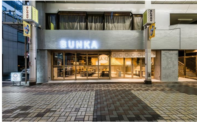
Figura 20_ Albergue Bunka - Fachada principal
