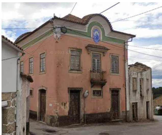
Figura 17 - Moradia "Bushell" (Google Maps, 2021).
